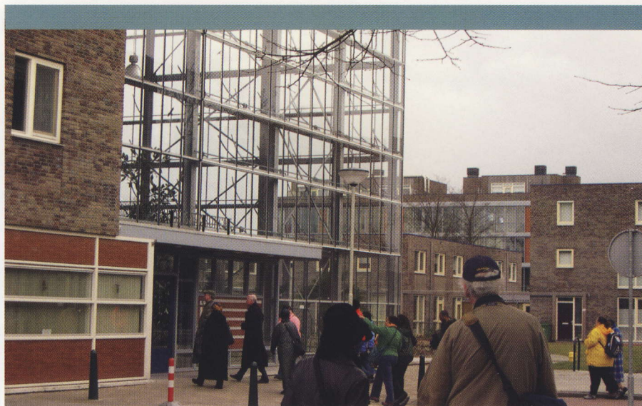
This new senior complex in Hoogvliet, a post-WW II social development under reconstruction outside Rotterdam, features a glass atrium with panels that open in summer.
