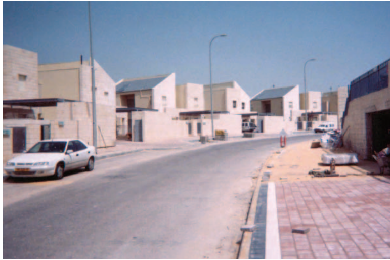
These homes are typical privately-financed houses in the new city of Modi'in. Their approximate average price is $300,000.
