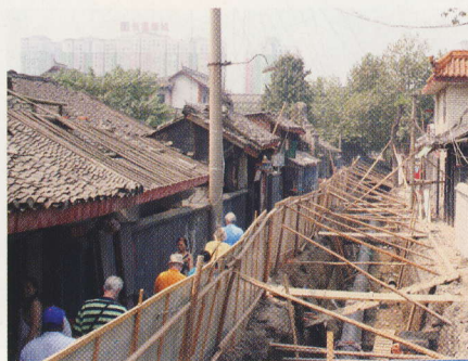
A sewer line installation in one of Chengdu's historic preservation areas.
