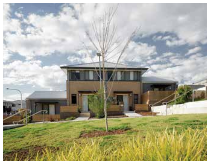
This project by Kennedy Associates features six dwellings, including two fully accessible single-storey units, two double-storey units and two 'Fonzie' flats above the rear garages. It was designed to house people with a disability and their extended family and/or carers Photo by Ben Guthrie
