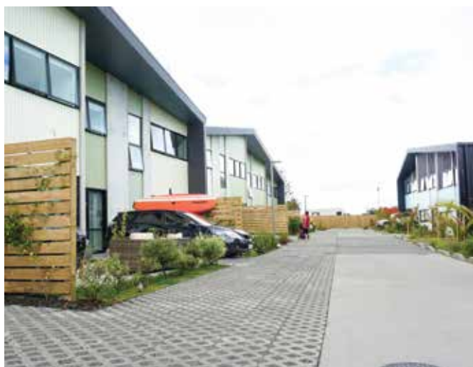
Swales and permeable paving treat stormwater run-off on-site, promoting kaitiakitanga (sustainable management) of water resources.
